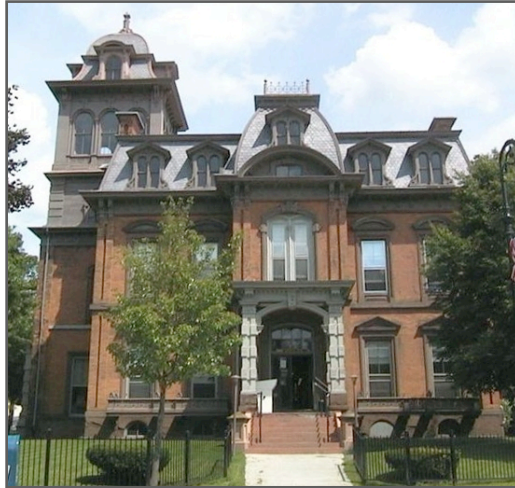
The North Adams Public Library is a model of green building design and the public face of Take Charge.
